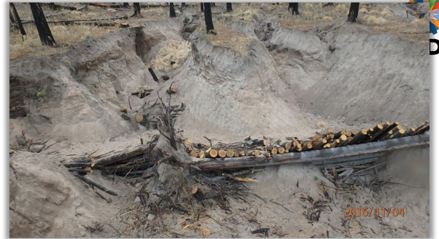
Headcutting Erosion Control Measure
