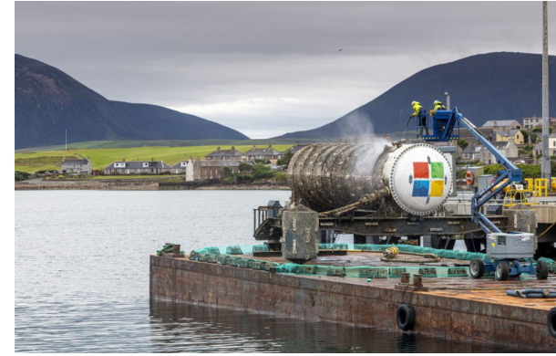
Data Centers and Energy Corridors
