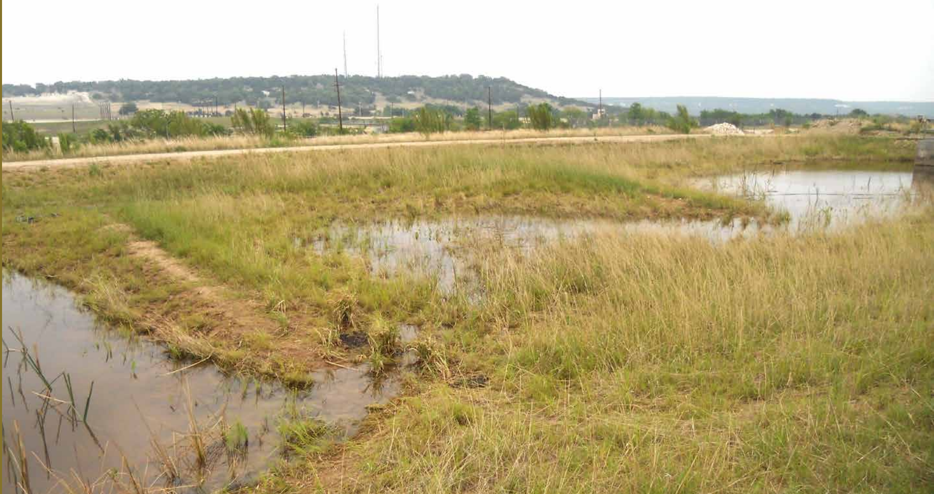
Below: A series of retention cells in the constructed wetland. (Photo by ERDC)
