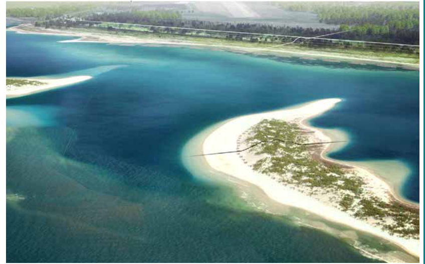
Above: For protecting inland assets from coastal flooding, nature-based solutions include enhanced sand trapping on the barrier islands and dune construction along the mainland. (Photo by Jacobs)
