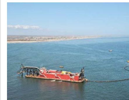
Dredge TEXAS working off of Stone Harbor, NJ for beach nourishment
